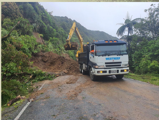
Above: Lisa at work with her team (right) and clearing flood gorge slip (left)
